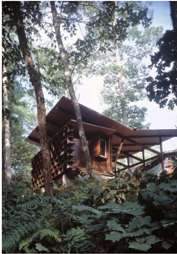
LEFT Southeast view of the Moore Honeyhouse (1998) in Cashiers, North Carolina, by Marlon Blackwell Architects.
